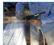
Intelaiature metalliche Metal framing
