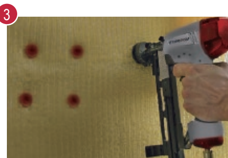
FS9240BC securing insulation layers
